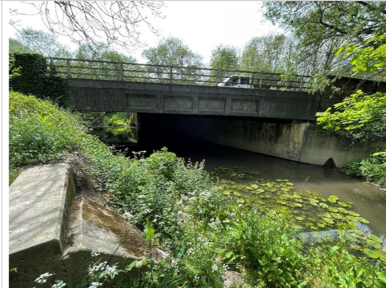
Photo 33: Downstream side of London Road bridge
