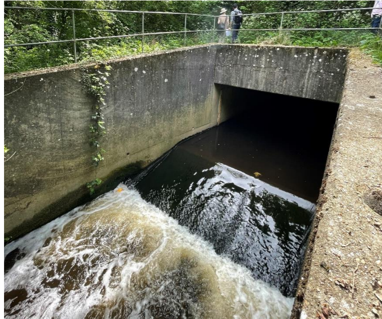
Photo 72: Airport Way culvert outlet and weir structure
