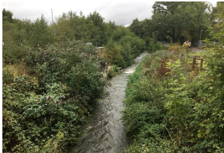
Photo 59: Run flow conditions, nick point in channel over step resulting in scour
