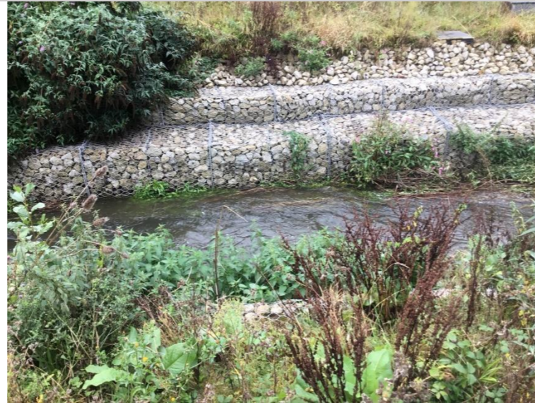
Photo 60: Gabion rock baskets provide bank protection on left bank due to scour at nick point in channel
