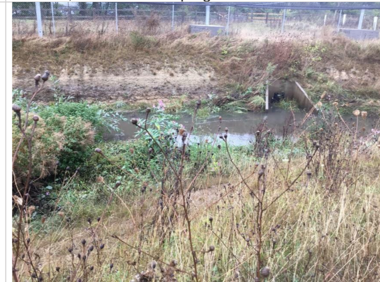
Photo 52: Outfall with concrete headwall on right bank
