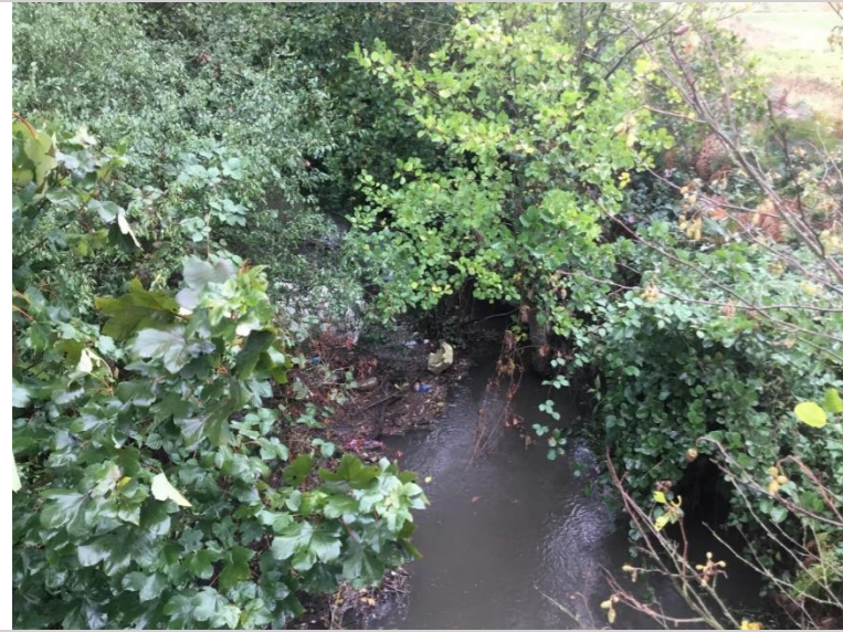
Photo 47: Rubbish accumulation at margins of channel
