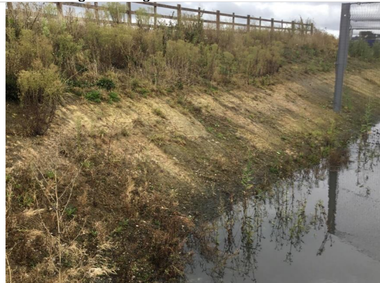
Photo 91: Geotextile over clay banks exposed
