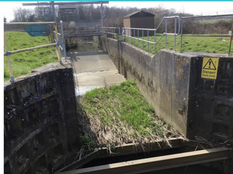
Photo 2: Syphon channel from River Mole and gravel accumulation next to drop chamber
