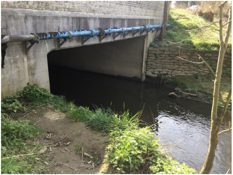
Photo 38: Downstream side of Brighton Road bridge
