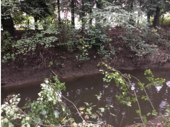
Photo 4: Over-steepened banks along straightened section
