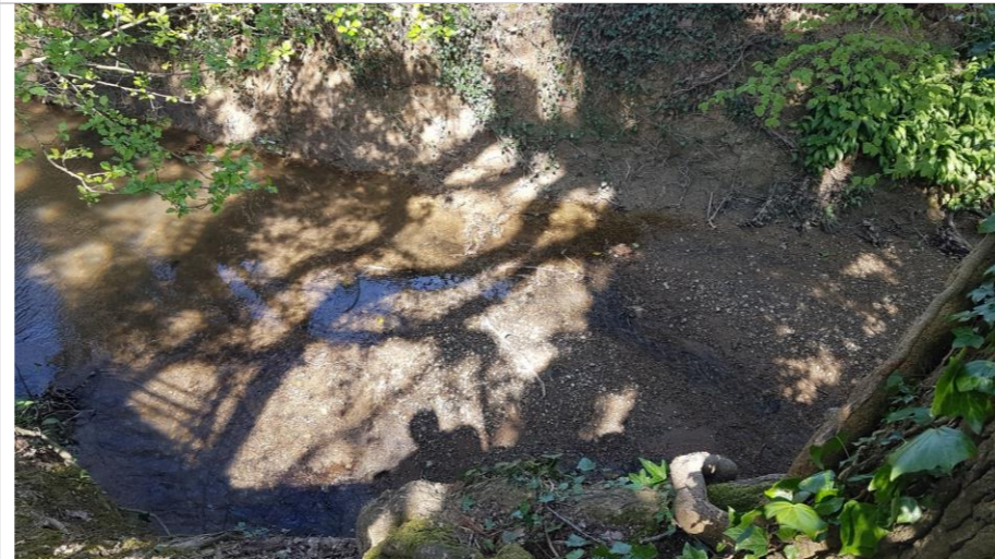
Photo 133: Localised widening of channel and notable deposits of fine gravel and silt creating low flow channel
