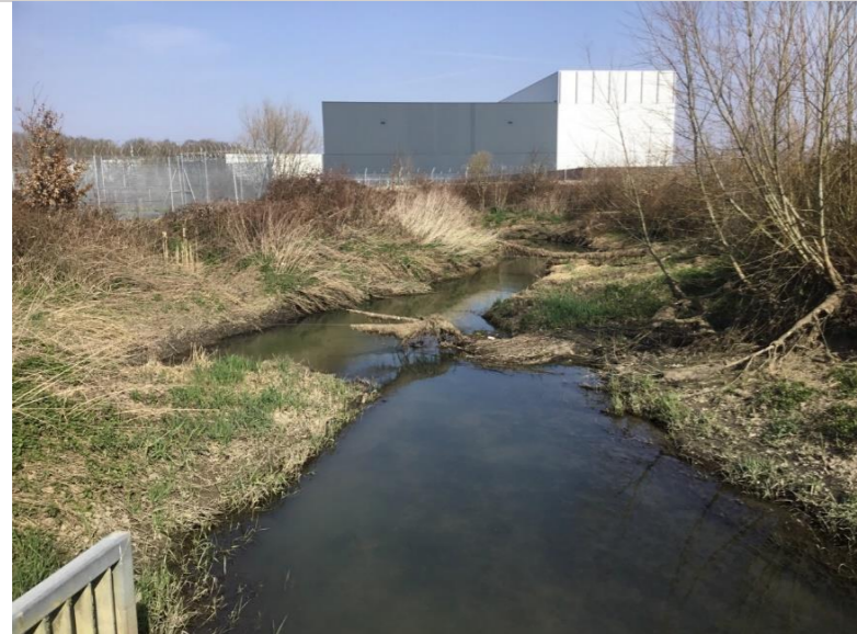
Photo 10: Downstream view of runway culvert outlet, channel is notably wide
