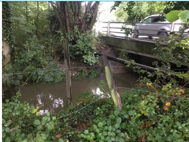
Photo 44: Radford Road bridge at furthest upstream extent
