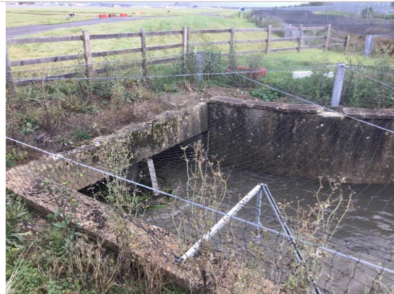
Photo 7: Runway box culvert inlet and divider wall
