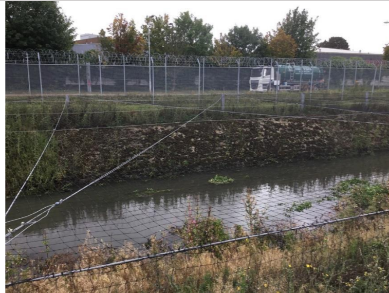
Photo 89: Concrete blockwork bank exposed on left bank
