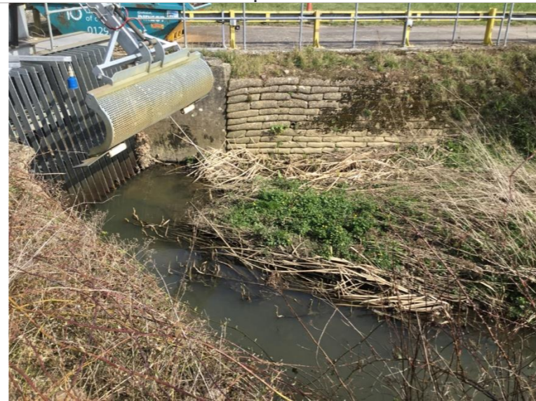
Photo 5: Weir structure upstream of culvert
