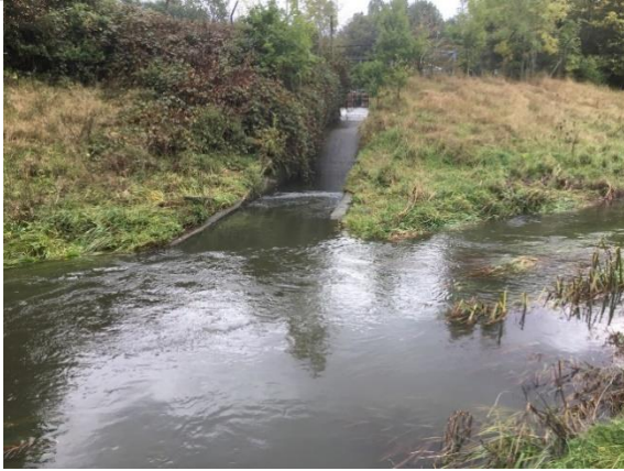
Photo 3: Concrete lined outfall structure set into the right bank
