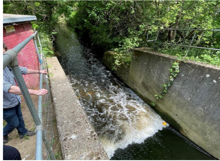
Photo 73: Downstream of Airport Way culvert
