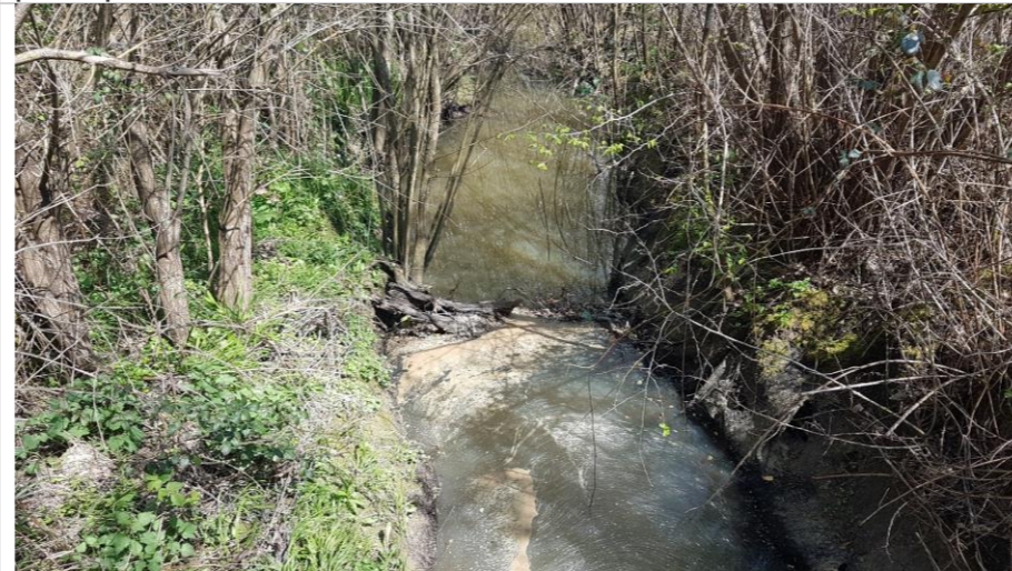
Photo 139: Small wood dam impounding flow. Lower bank top height. Heavily shaded.
