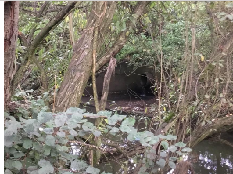
Photo 32: Outfall on right bank upstream of London Road bridge, concrete headwall
