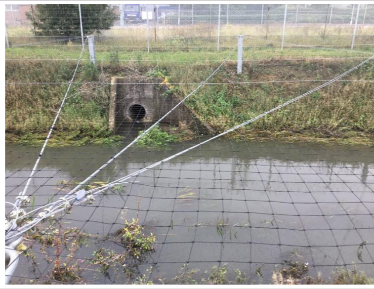
Photo 101: Concrete outfall on left bank
