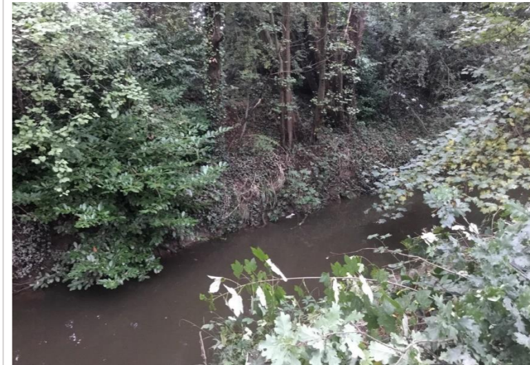
Photo 83: Steep heavily vegetated banks along straightened section of Gatwick Stream approaching confluence with River Mole
