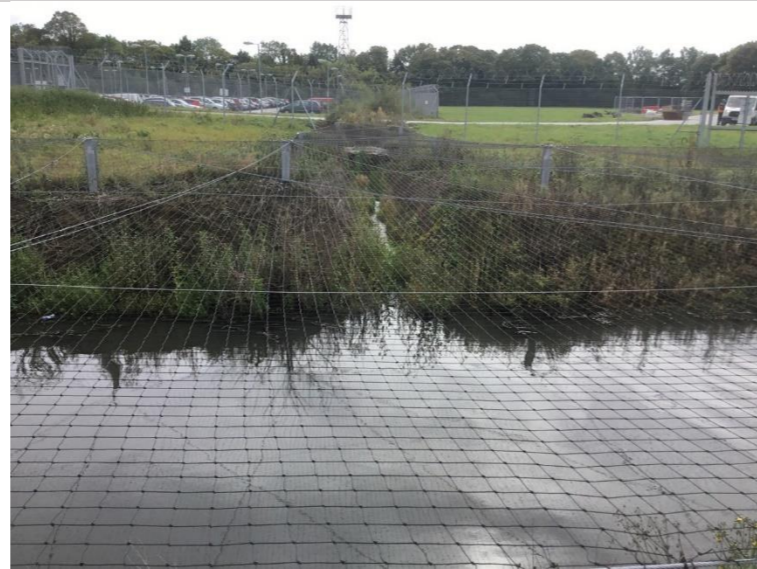
Photo 110: Concrete outfall and spillway on left bank at Car Park X
