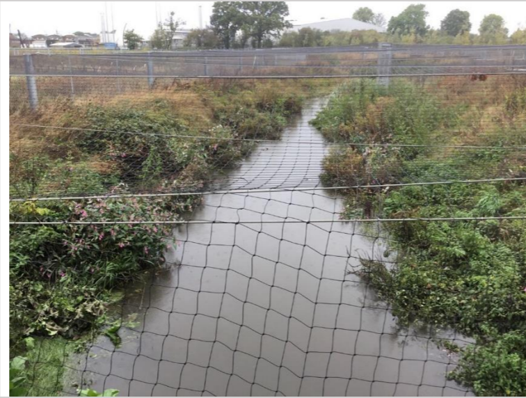
Photo 48: Netting over channel within Gatwick Stream biodiversity area
