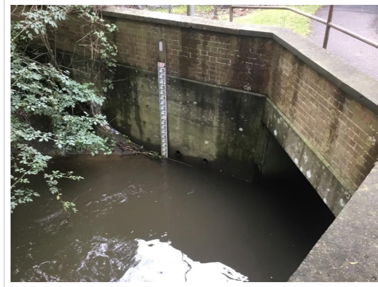
Photo 68: South Terminal culvert outlet
