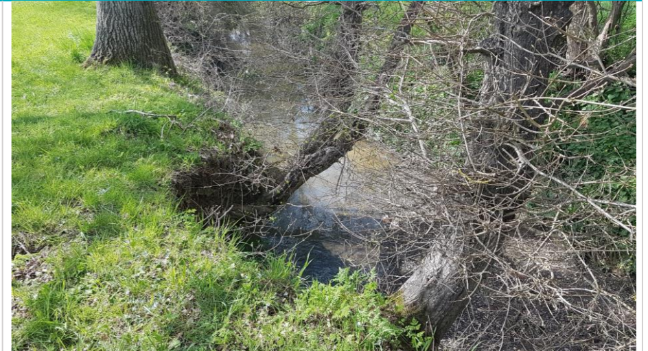
Photo 119: Undercutting of bank opposite gravel bar, overhanging trees
