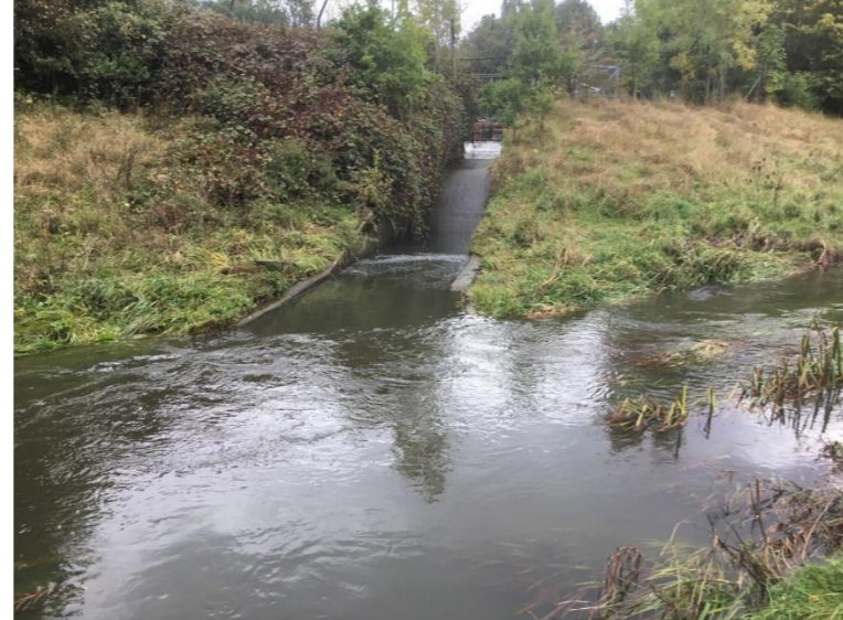
Photo 29: Concrete outfall from Pond D
