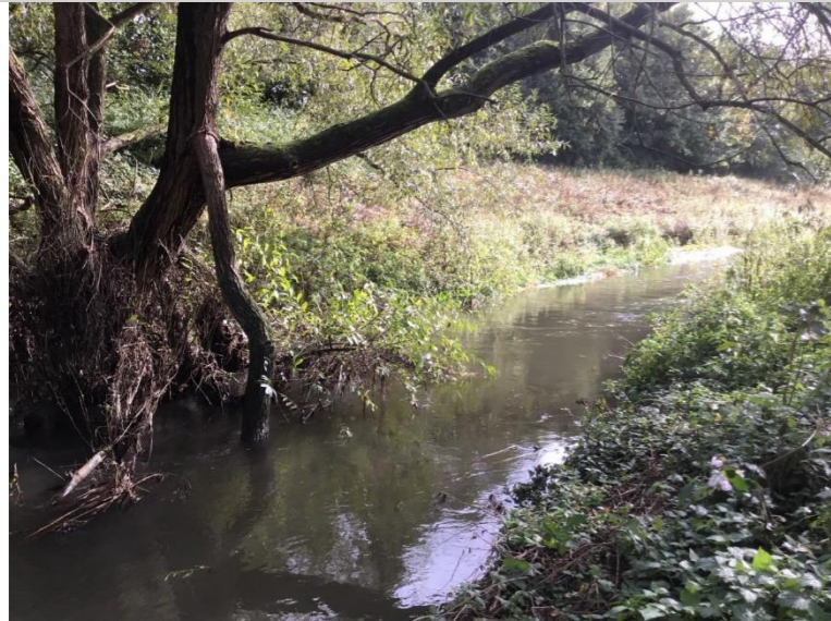
Photo 31: Approach to London Road bridge, roots submerged in channel
