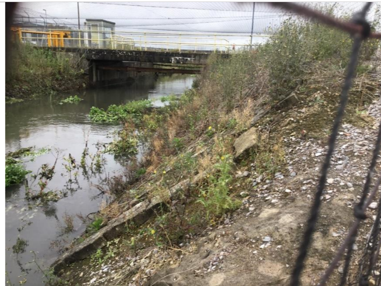
Photo 92: Concrete blockwork on right bank
