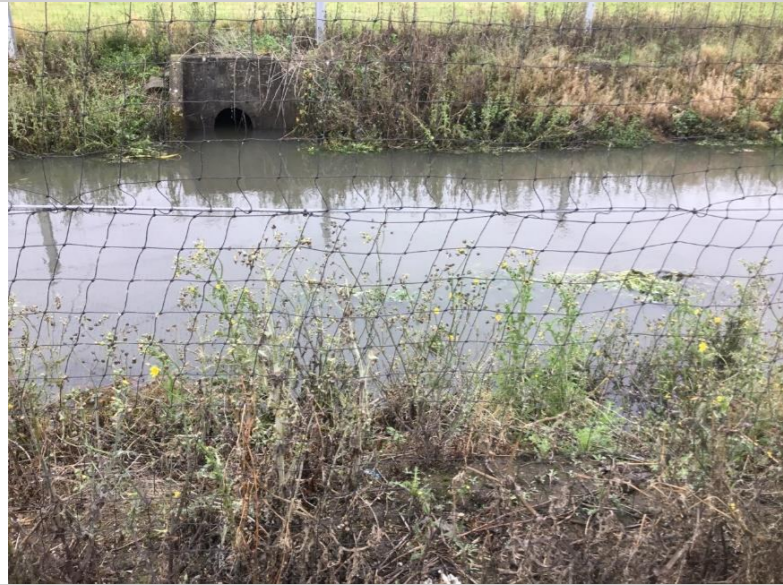
Photo 100: Concrete outfall on left bank
