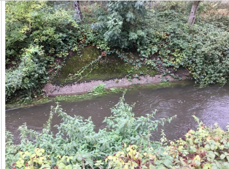
Photo 58: Channel is concrete lined from railway bridge downstream along straightened section to footpath bridge
