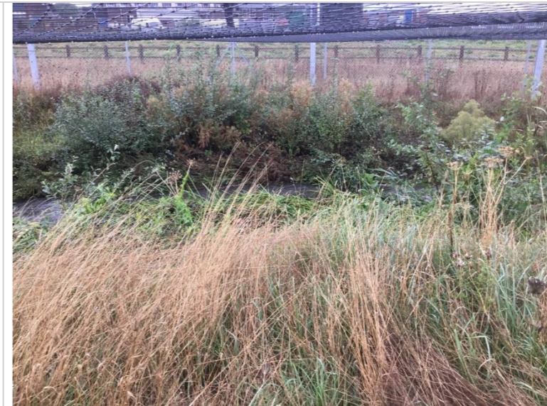
Photo 55: Narrow section of channel resulting in increased velocities
